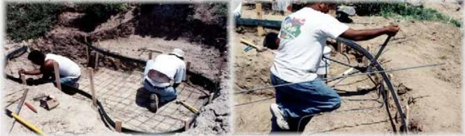
After the pond is excavated, a laser level is used to level the green bender board forms to establish the level of the ponds perimeter. Stakes are placed and marked first and the board screwed to
