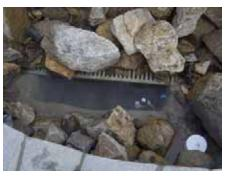
Collection basin containing the anti-vortex drain and AquaFill electronic auto level float control system.
