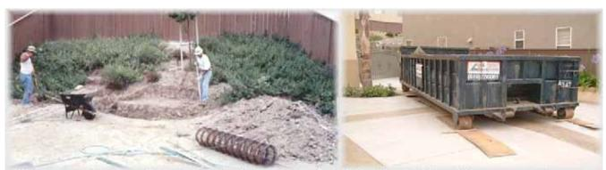
When excavating a pond in a backyard with no access for a Bobcat or backhoe, it is necessary to remove the dirt by hand and transport it to a dumpster in front, using a wheelbarrow and a plank for a ramp.
