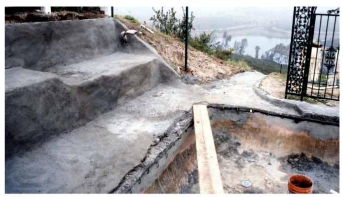
**Above:** The fence was temporarily removed during construction to create an exit stream that appears to be running over the edge of the hill on its way to the lake below. However, the stream actually ends just over the crest of the hill, spilling into a screen covered well which collects the water. A submersible pump directs the collected water back to the pond.
