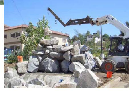
nature to see that they never are made up entirely of small, uniform cobble rock. The majority of rocks in a waterfall created by nature are huge in using a crane to set a few large rocks. Cranes can cost \$100-\$200 per hour, depending on the size, plus a move-on fee and travel time. A couple of hours of crane time and approximately \$600 worth of boulders and trucking will make an difference in the finished project.
