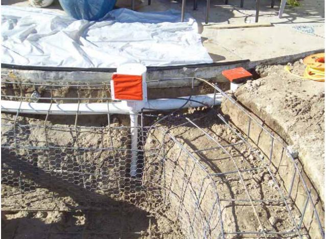
Skimmer and overflow drain for pond just prior to pumping concrete.
