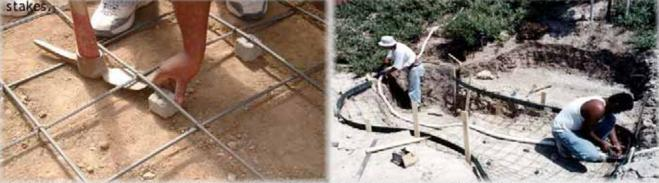
Dobie blocks are used to hold the rebar off the ground so the concrete will totally encase it. Also, flexible PVC pipe can run between the rebar and ground in the two inch clearance provided by the blocks.
